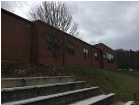
4). North Elevation - Feb 02, 2017
