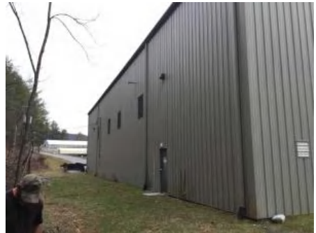
3). Northeast Elevation - Feb 01, 2017
