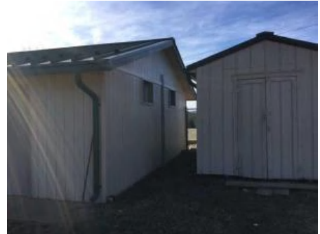
3). North Elevation - Feb 01, 2017
