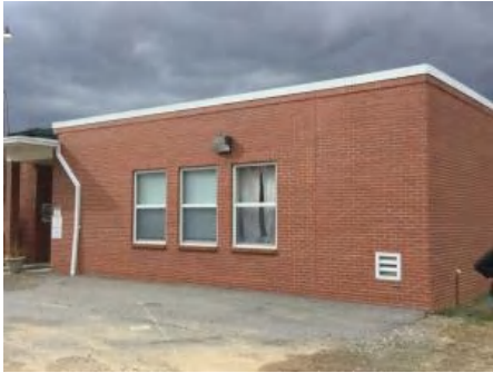
1). East Elevation - Feb 01, 2017
