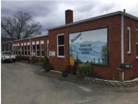
1). South Elevation - Feb 01, 2017
