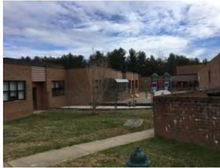
2). South Elevation - Feb 01, 2017
