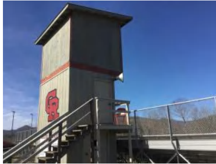
2). Southeast Elevation - Feb 02, 2017
