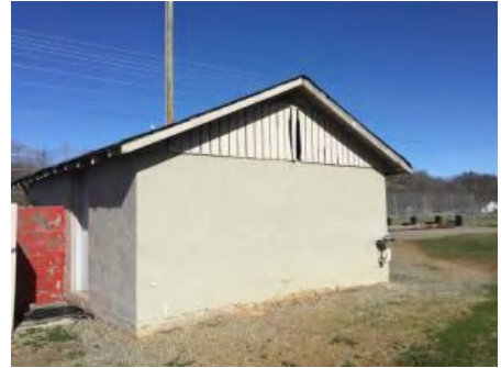
3). South Elevation - Feb 02, 2017
