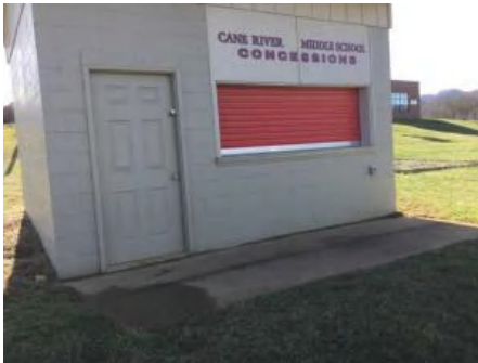
1). North Elevation - Feb 02, 2017
