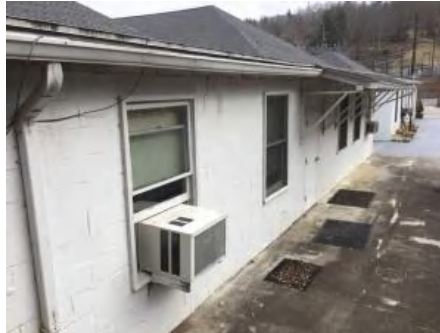
2). South Elevation - Feb 01, 2017
