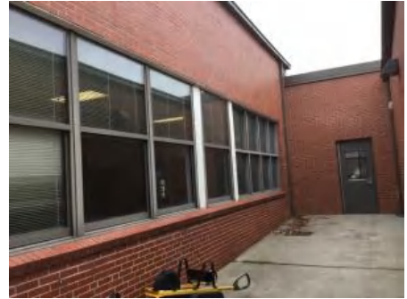
3). South Elevation - Feb 02, 2017
