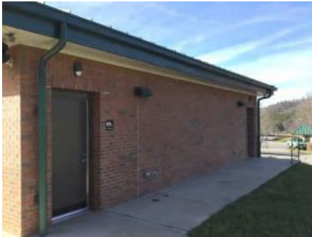
4). Southeast Elevation - Feb 01, 2017
