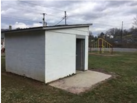
1). South Elevation - Feb 01, 2017
