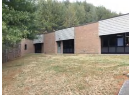
3). South Elevation - Feb 01, 2017
