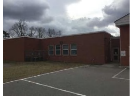
3). North Elevation - Feb 01, 2017
