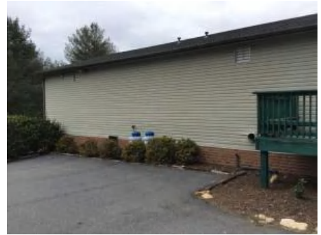
3). South Elevation - Feb 01, 2017
