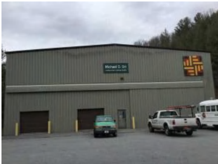
1). Southeast Elevation - Feb 01, 2017
