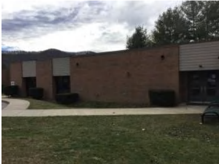
1). North Elevation - Feb 01, 2017
