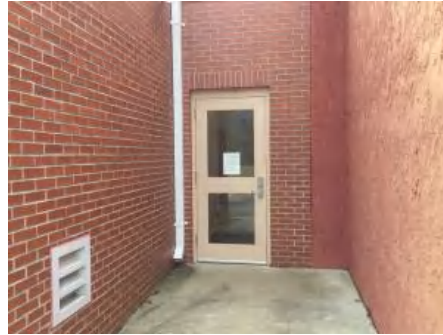
2). North Elevation - Feb 01, 2017
