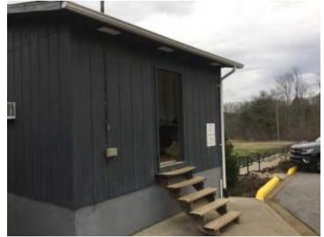
3). South Elevation - Feb 02, 2017
