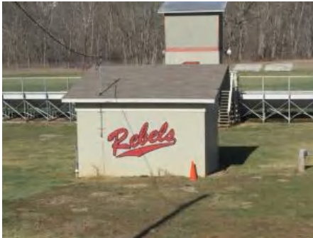
4). South Elevation - Feb 02, 2017
