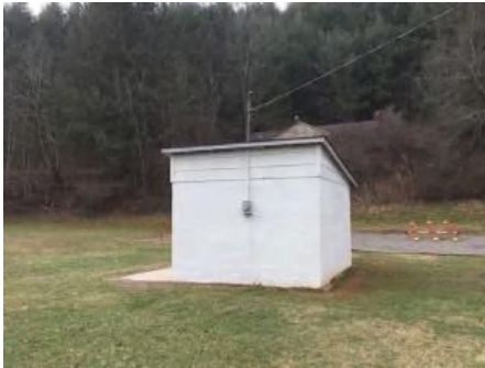
4). North Elevation - Feb 01, 2017
