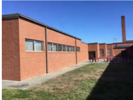
2). South Elevation - Feb 02, 2017
