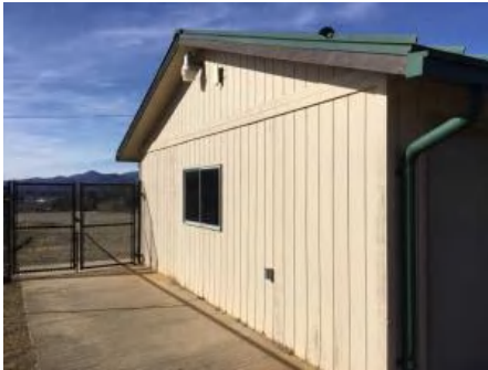
4). South Elevation - Feb 01, 2017
