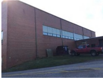
2). North Elevation - Feb 02, 2017
