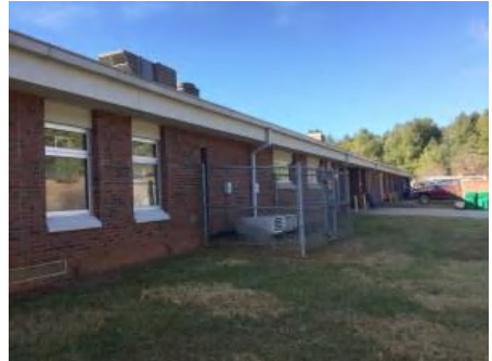
3). North Elevation - Feb 01, 2017
