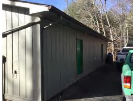
2). East Elevation - Feb 01, 2017
