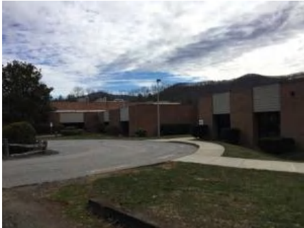
1). North Elevation - Feb 01, 2017
