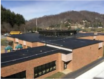
1). Northeast Elevation - Feb 01, 2017
