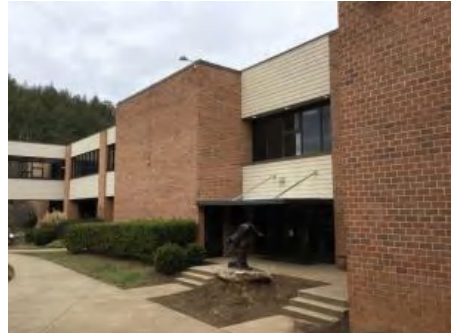
3). South Elevation - Feb 01, 2017
