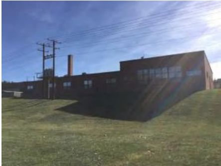
1). North Elevation - Feb 02, 2017
