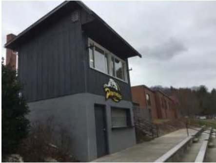
1). North Elevation - Feb 02, 2017
