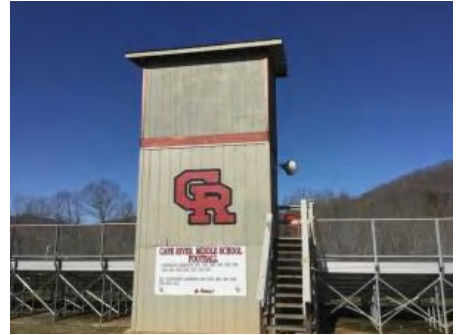
3). South Elevation - Feb 02, 2017
