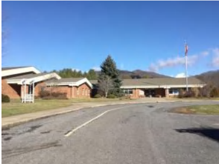
1). South Elevation - Feb 01, 2017
