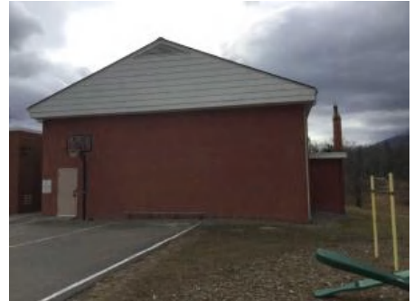
3). North Elevation - Feb 01, 2017
