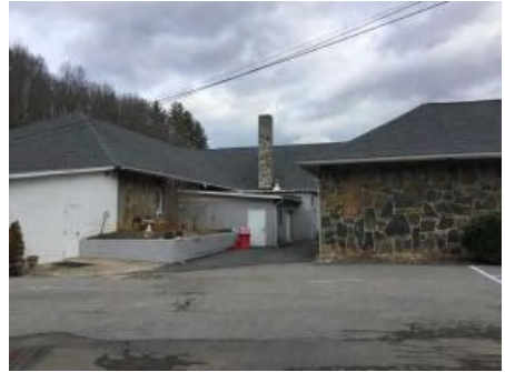
3). South Elevation - Feb 01, 2017
