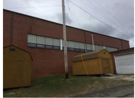
3). North Elevation - Feb 02, 2017
