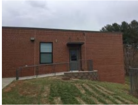
2). East Elevation - Feb 02, 2017
