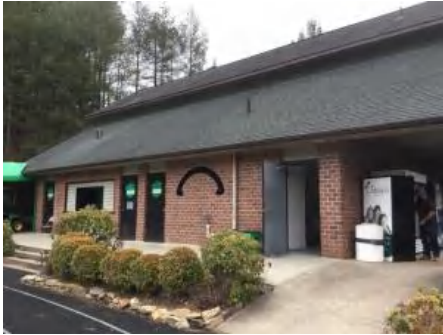
1). North Elevation - Feb 01, 2017
