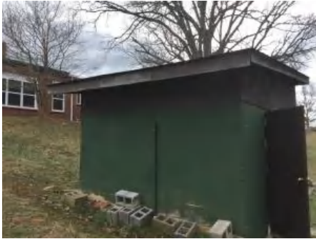
1). North Elevation - Feb 01, 2017
