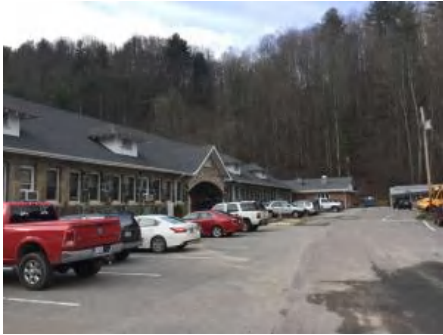
1). North Elevation - Feb 01, 2017
